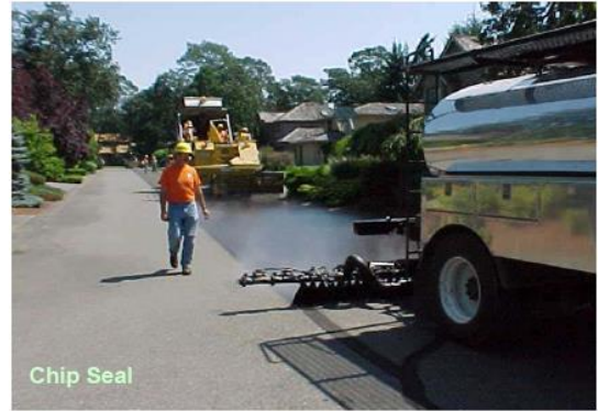
Photo shows work being done to preserve a Pierce County roadway.
